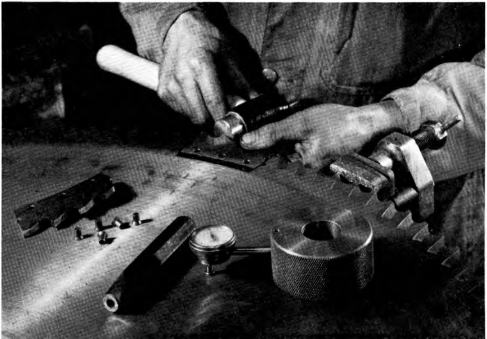
82. Fitting high-speed steel segments to a metal-cutting cold saw
